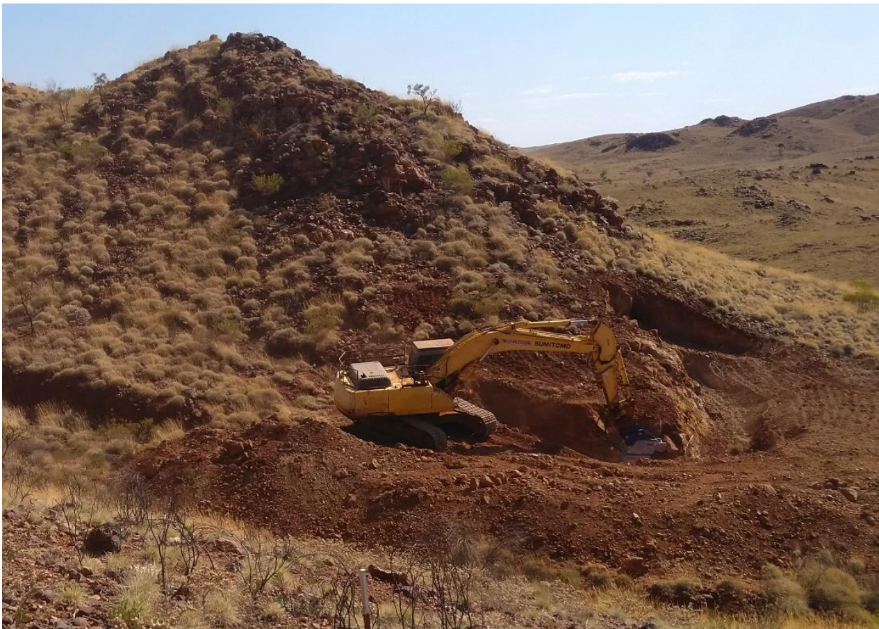
Figure 1 Trenching commences at Loudens West with Excavator on site
