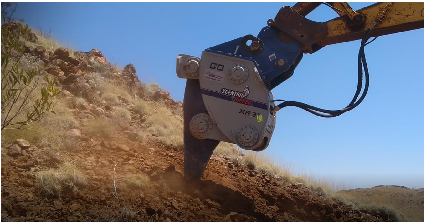
Figure 2 Xcentric Ripper being used at Loudens
